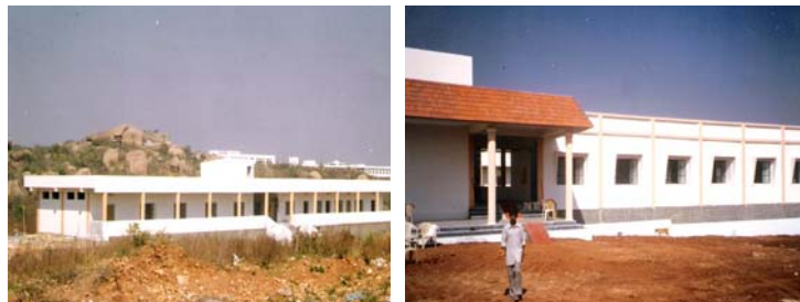
Buildings constructed for Department of Publications and Men's Hostel not put to use
