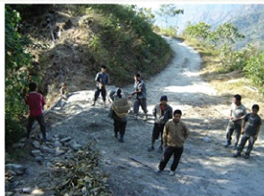
Village road to aid in rural connectivity at Jarong, South Sikkim
