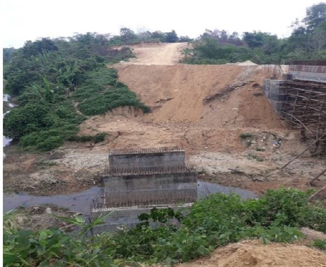
Construction of three abutment walls in middle of Rubri Cherra under Hezamara Sub-Zone
