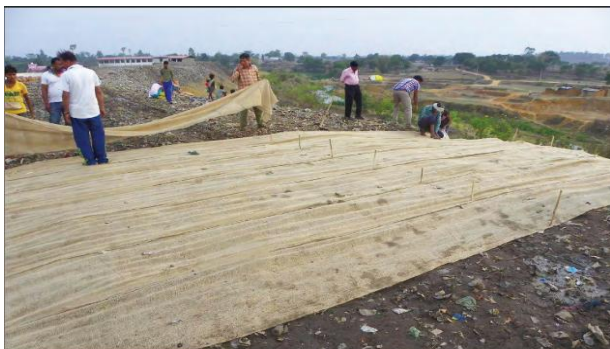
Figure 2 Ambikapur Legacy waste treatment: Jute capping, after which the entire waste surface is covered with capping materials like leaf
