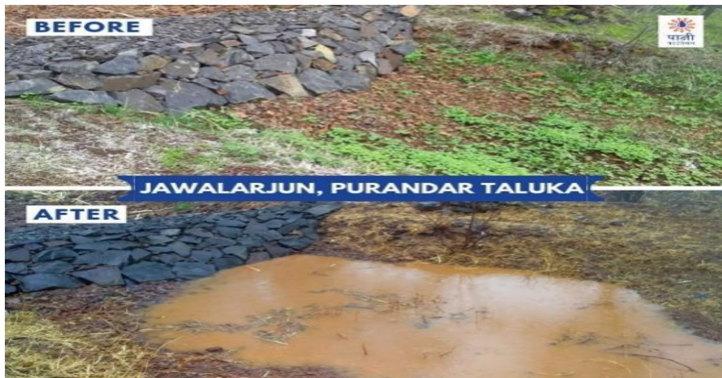
Figure 11 (a) Earthen Nala Bund at Jawalarjun, Source- Panni Foundation, Satyamev Jayate (2019) (instagram, n.d.)
