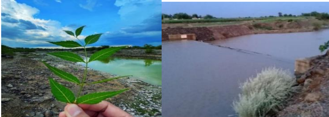
Figure 13 (a) CNB Structure on Karha River (Before and After) structure 3
