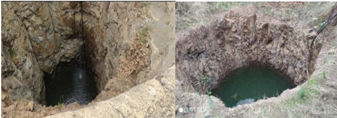
Figure 13 (b) Water level (Before and After) in nearest the well of CNB structure at Jawalarjun village (Green Foundation, n.d.)
