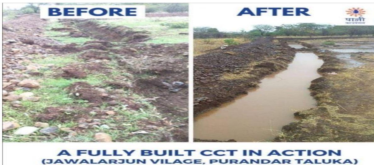
Figure 12 Continuous contour Trenching (CCT) in Jawalarjun Village, Source- Panni Foundation, Satyamev Jayate (2019 (Facebook, 2019) )
