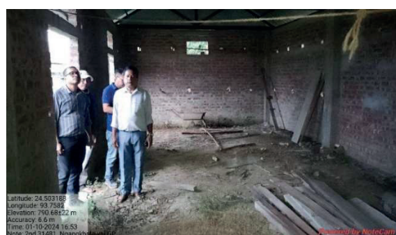
Inside the building of AWC at Ngangkhalawai GP
