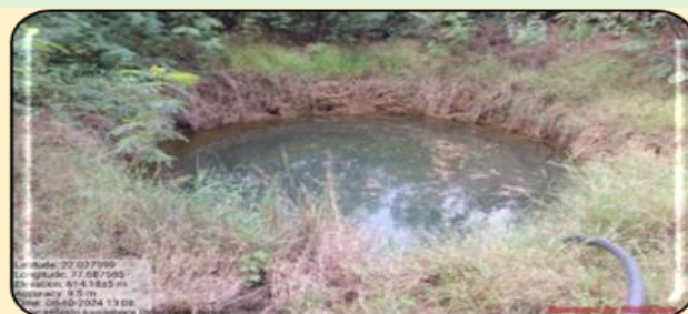
Pic 6.10: Picture taken during JPV, shows the absence of the required RCC ring wall around the Kapil Dhara Koop, as mandated by the guidelines issued by PRDD, GoMP (May 2019). Further, the construction was to be completed within one year from the date of sanction. However, despite an expenditure of ₹1.54 lakh, the work remained incomplete even after six years of sanction.
