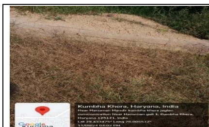
Photograph No. 2.7: Work of desilting and digging of pond near vayamshala
