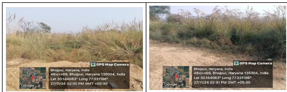
Photograph No. 2.4 and 2.5: Work of land levelling on Panchayati land, GP Bhojpur Parwalo
