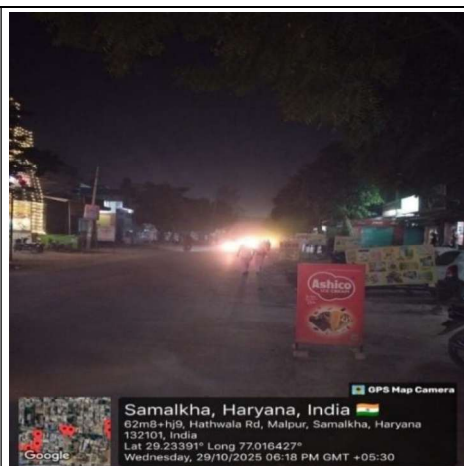
Photograph 1 : exhibiting no streetlights at Hathwala Main Road
