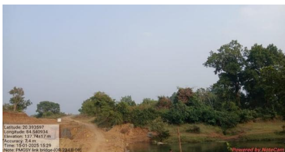
Picture 3.2.3: HL Bridge on RD road at Ambalimba (Date: 15 January 2025)
