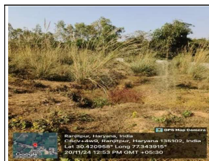
Photograph No. 2.8: Work of earth filling on Panchayati Land at GP Sultanpur
