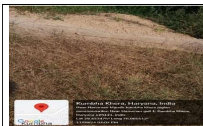
Photograph No. 2.7: Work of desilting and digging of pond near vayamshala
