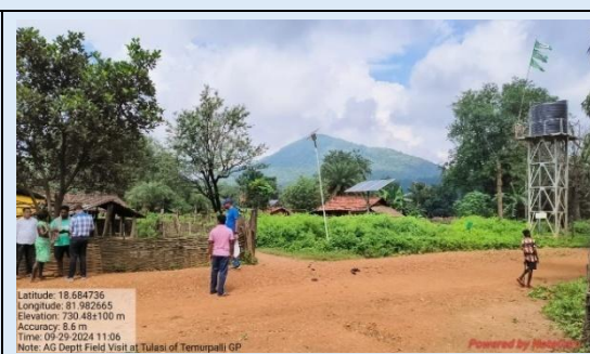
Photo 2: Solar energy-based water supply system at Tulasi village of the Mathili Block (118 HHs) (29 September 2024)
