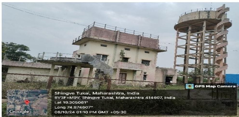
Photograph 1: Unused WTP and ESR in Shingve Tukai village (Ahilyanagar district)
