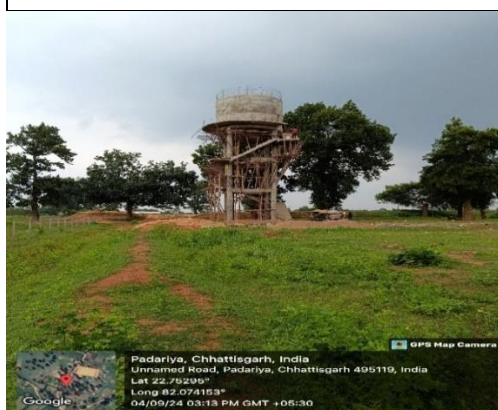
Photo 4.10: Incomplete OHT at village Padariya, District: GPM
