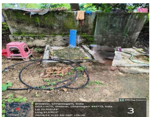
Photo 4.5: Picture showing FHTCs at village Bhidavar with composite pipe not connected with distribution line
