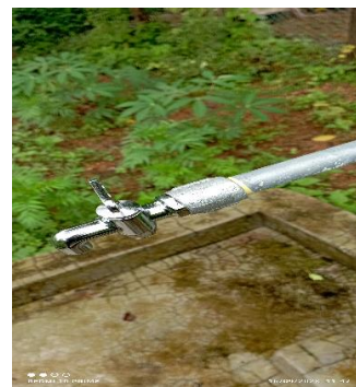
Photo 3.2: Picture showing 15mm taps being used in FHTC
