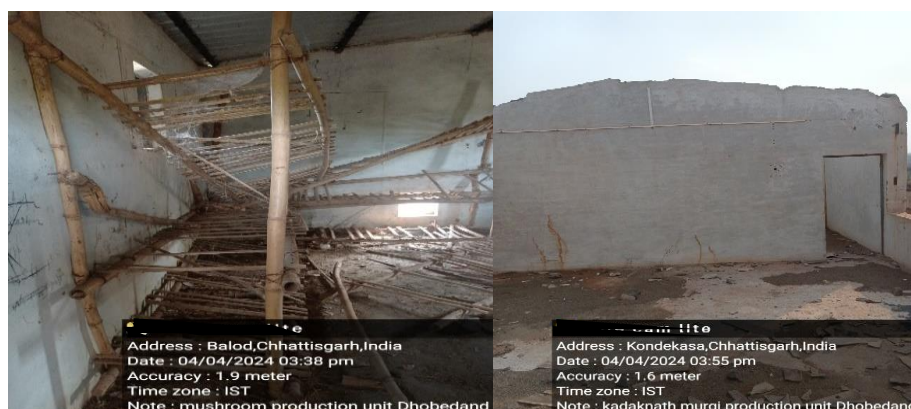
Picture 3.8: Photos of Poultry and Mushroom Production Centres established from DMFT funds in Janpad Panchayat, Dondi
