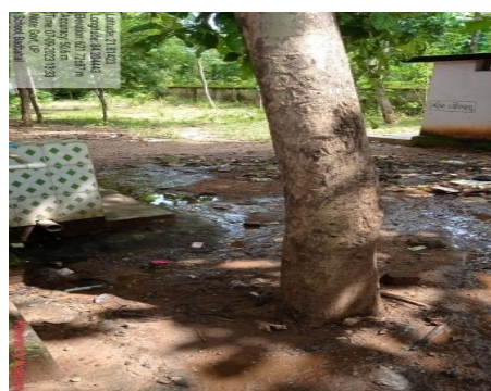
Photograph 14: UPS, Badbahal: No drainage facility available
