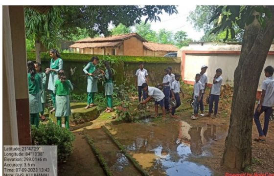
Photograph 13: GHS, Kulihamal: No drainage facility available
