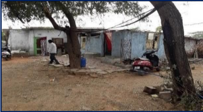
Picture 6.4: Encroachments on Praga Tools land
