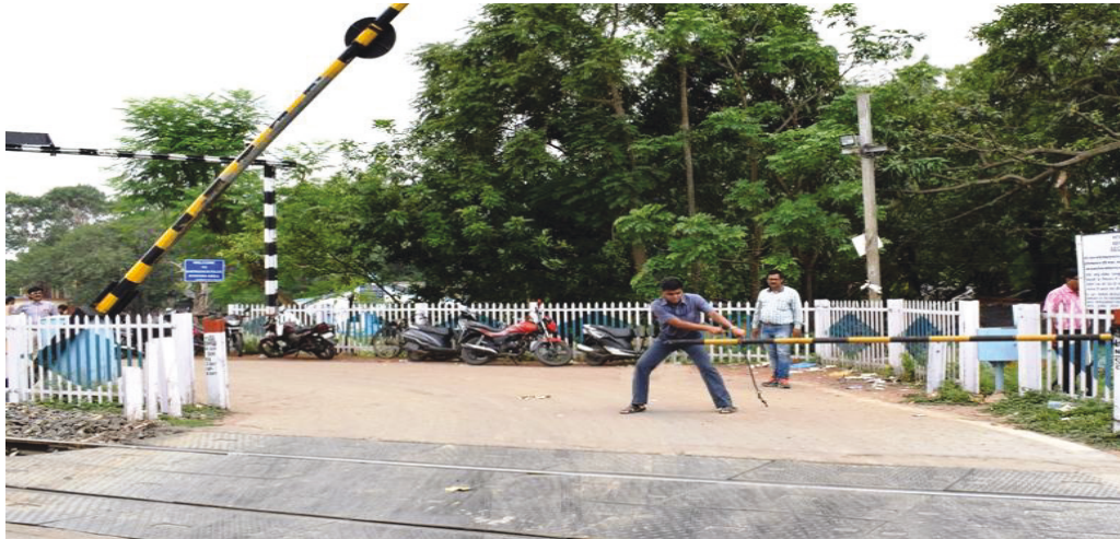
Image 2.1: Emergency Sliding Booms
