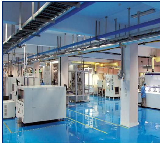
Figure 4.4: 85 MW Solar Cell Manufacturing Facility
