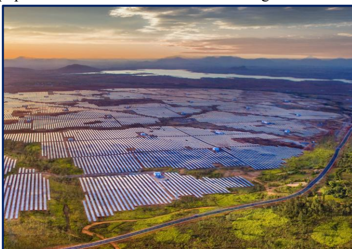
Figure 4.1 - Kadiri Solar Park, Sri Satya Sai District, Andhra Pradesh
