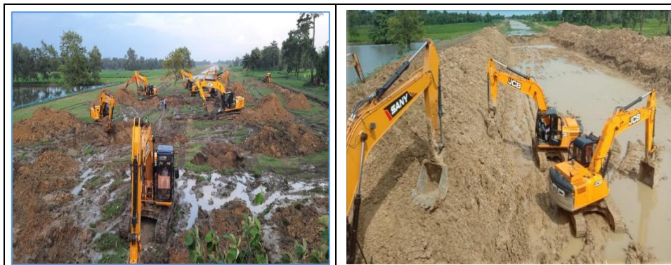
Photograph-3.1: Digging of RMC at Laxminagar, Balrampur using hydraulic excavators (Poclain machines)
