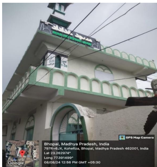
Photograph 3.4.1: Religious building constructed in the land registered as waqf in Sanjay Nagar, Bhopal (Picture taken during joint survey dated 8 August 2024)
