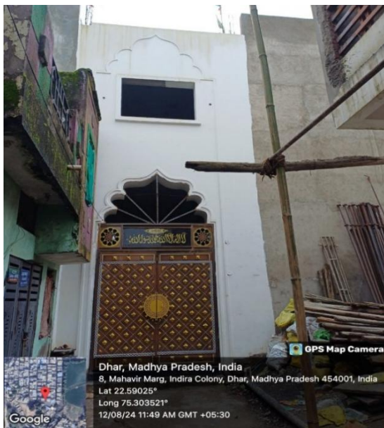
Photograph 3.4.3: Waqf property registered without clear title of ownership at Islampura, Dhar (Picture taken during joint survey dated 12 August 2024)
