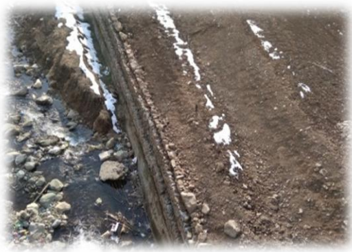
Spot work done inside the Saidnar nallah thereby reducing the width of the nallah from 100-150 feet to 25 – 30 feet
