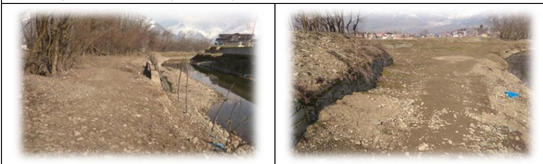
Extracted material dumped at the Lake fringe resulting in shrinkage of nallah
