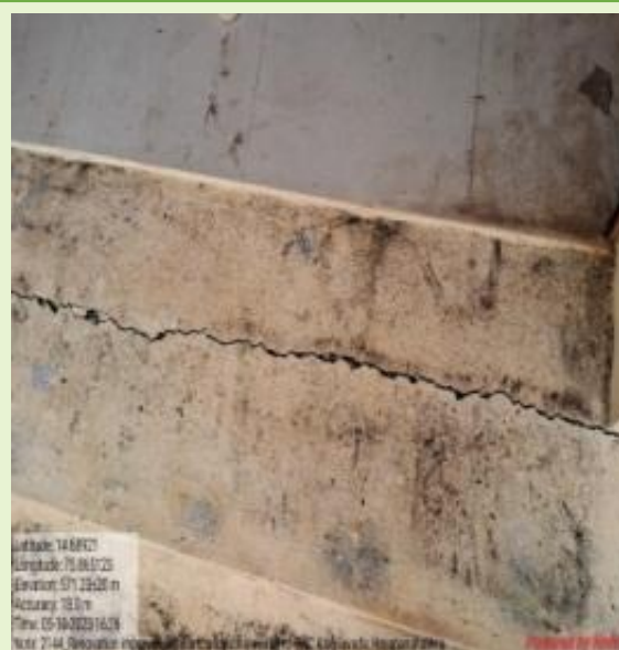
Picture No. 5.12: Cracks in the building repaired through Nirmithi Kendra at PHC Alagilawada, Harappanahalli.
