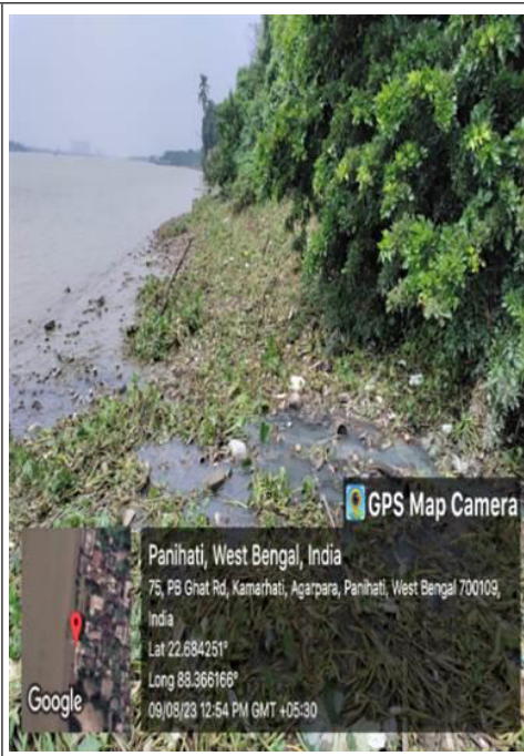
Figure 4.2: PB Ghat drain falling into Ganga untapped.
