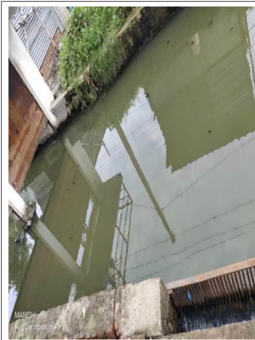
Figure 4.1: A portion of the sewage from nearby drain was being taken to the pumping station for feeding STP.
