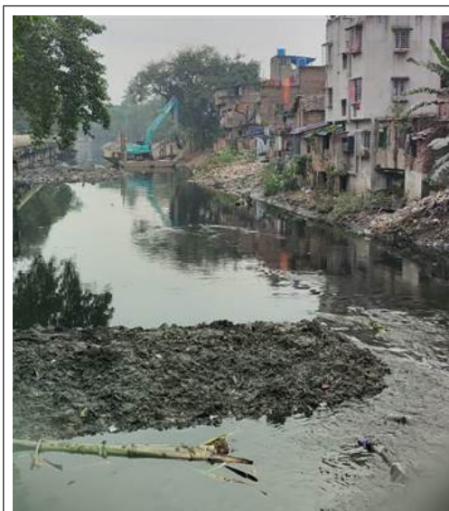
Figure 4.12: Dredging work in progress
