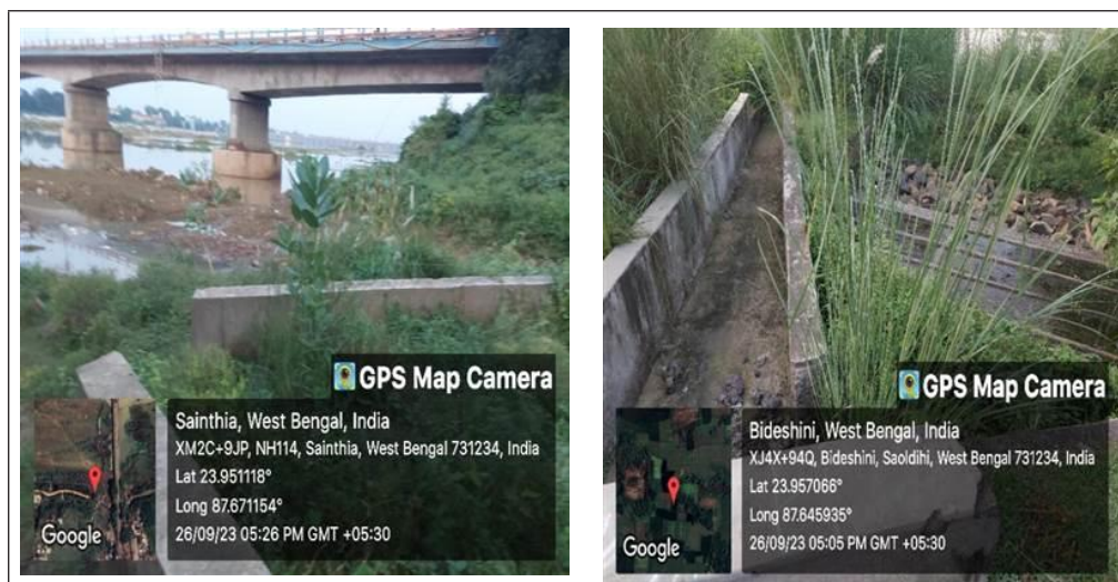
Figure 4.21 : In-complete bio-remediation works for treatment of drain water at Sainthia
