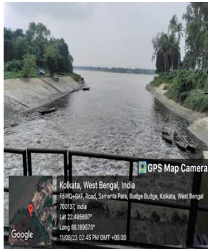
Figure 4.6: Churial drain discharging in River Ganga.
