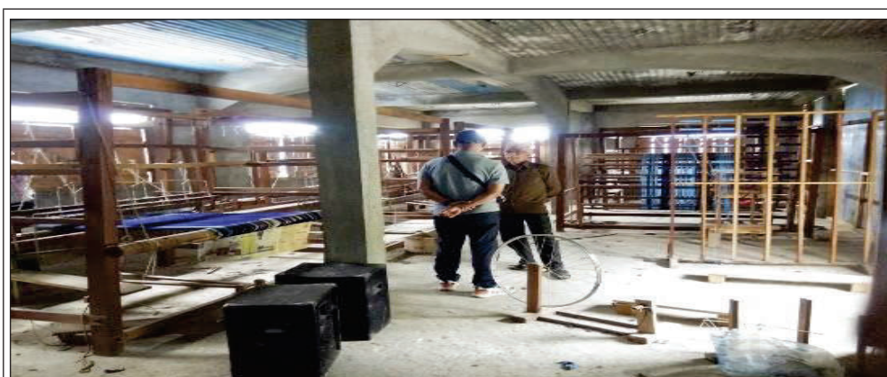
Fig. 4.7: Installed Looms at Kagey Centre
