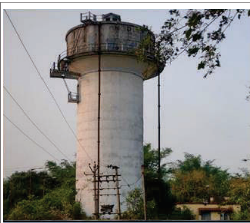
Fig. 4.13: Deserted Over Head Reservoir and Pump House-I, dated 21.05.2023
