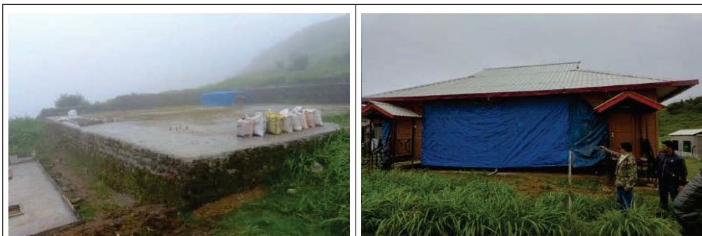
Fig. 3.4: Under construction cottages at Tonglu, Darjeeling
