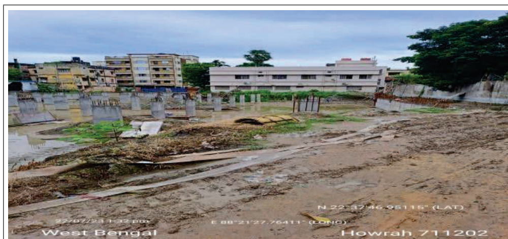
Fig. 3.21: Under construction car parking at Belur in Howrah
