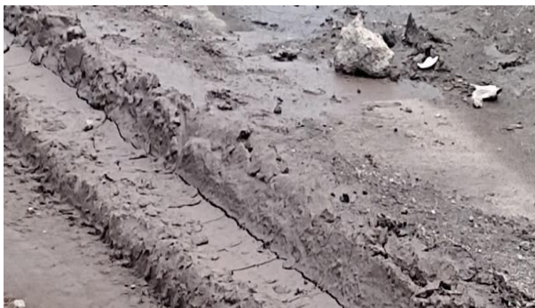
Photo No.30 - Gopalpur-Chhatisgarh Boarder Road
