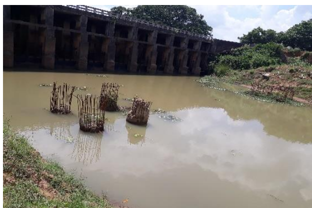
Photo No.27 - Bridge at chainage 5.080 km
