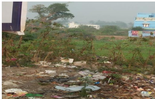
Photo No.31: Ucompleted portion of road and bridge of Khandia Bandha to NH by-pass (NH-316)
