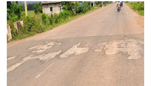
Photo No. 21: Pothole in SDBC on the roof slab of the box culvert
