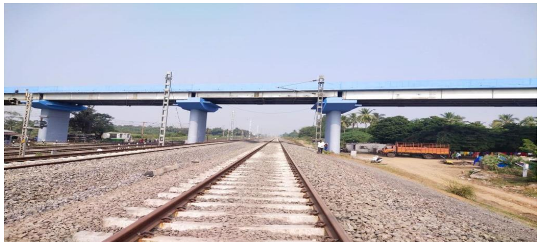
Photo No. 9: Rail Over Bridge
