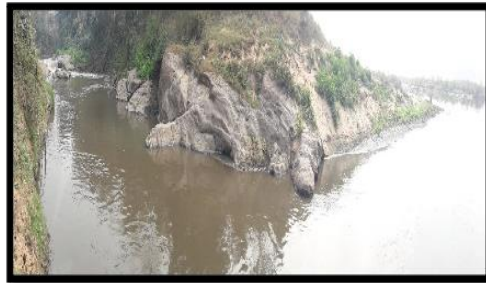
Photo No.1: River Brahmani at Tarkera Ghat
