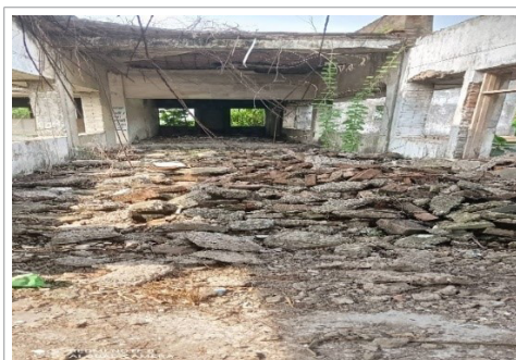
Images 6: Roof corridor of manufacturing plant of BVSL, at Industrial area, Hajipur (Vaishali)
