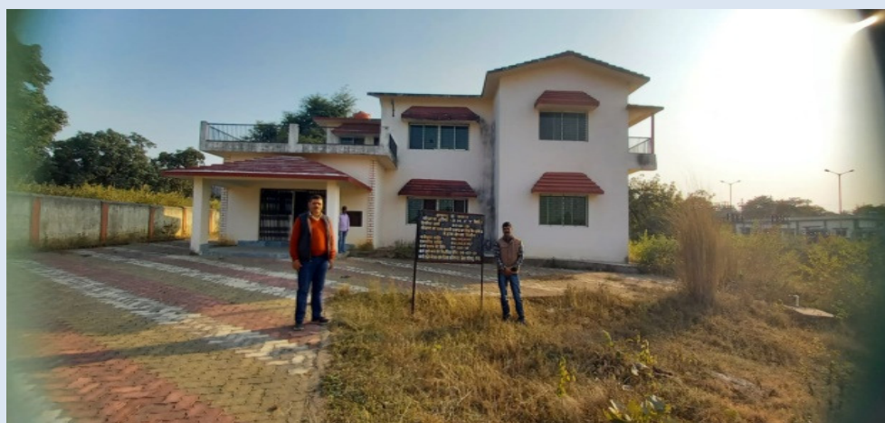
Picture 2: Dak-bungalow, McCluskieganj.
