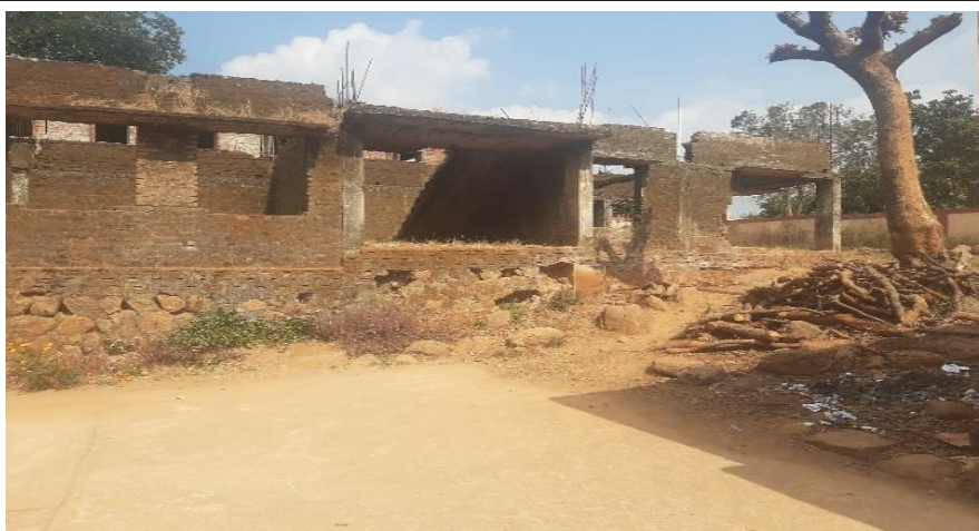
Photograph 3.1.1: Incomplete STGH building at Lubengarh, Th. Rampur, Kalahandi
