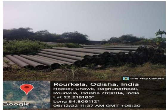
Photograph 28: Sewer pipes for Rourkela East Project, dumped at the project site, without utilisation
