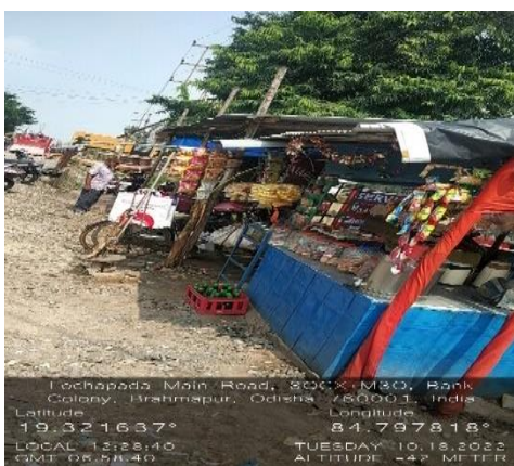
Photograph 31: Unauthorized construction of shop over the drain, near Dhobanallah,, Berhampur Municipal Corporation
