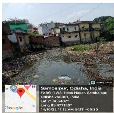
Photograph 32: Encroachment in the Dhubijore Nallah, Sambalpur
