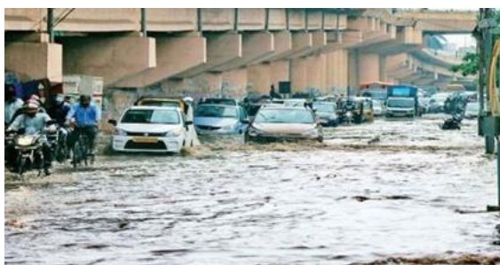
Photograph 1: Water logging at the Bomikhal flyover bridge, Bhubaneswar, e-Prameya (newspaper dated 27.09.2022)
