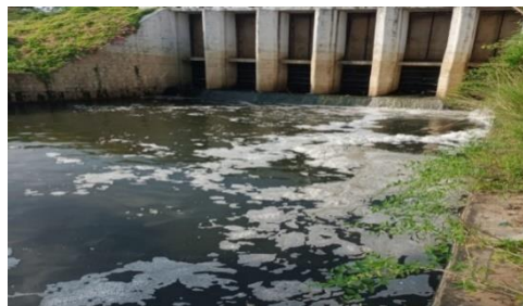
Photograph 27: Outfall of Dhobijore nallah into river Mahanadi, due to non-completion of the sewerage project
