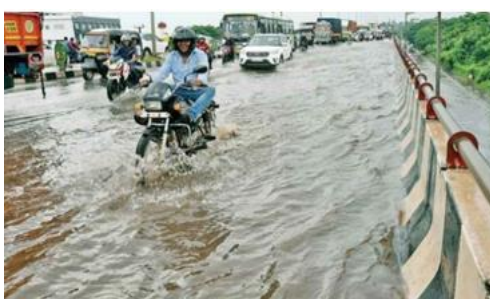
Photograph 2: Water logging at the Baramunda flyover, Bhubaneswar, e-Prameya (newspaper dated 27.09.2022)
