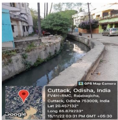
Photograph 23: Drain without cover slab near Rajabagicha Cuttack
