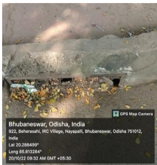
Photograph 9: Beherasahi road, IRC village PWD road, BMC
