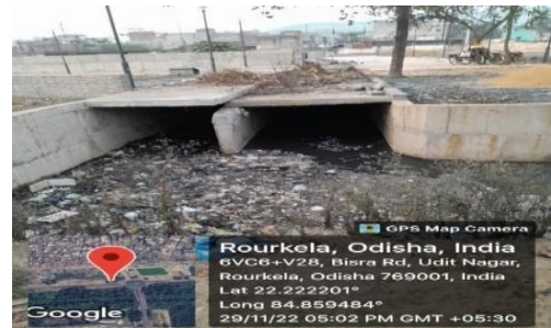
Photograph 43: Dumping of garbage in open drains, at the Bisra Road, Udit Nagar Rourkela
