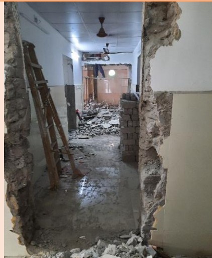
Modification work at the newly constructed SDH Building (10 May 2022)
