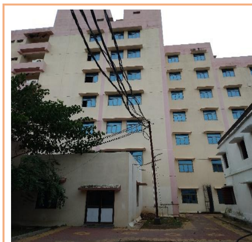
Laboratory complex at MKCG MCH, Berhampur (16 July 2022)
