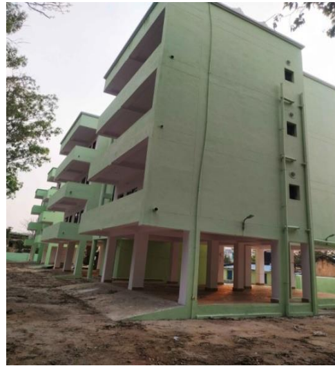
E-type quarters at DHH, Kandhamal, not handed over after completion (29 April 2022)
