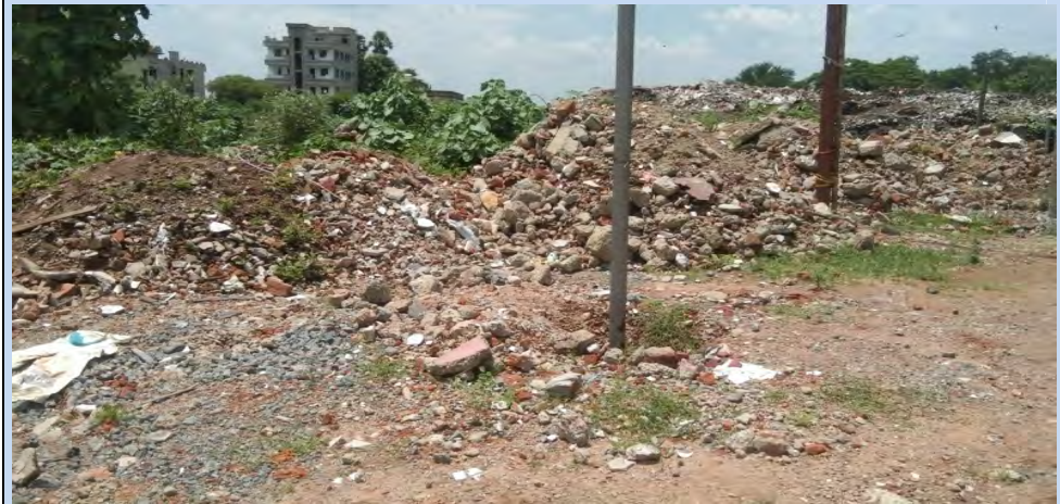
C&D waste lying on the road side, at the Medininagar Municipal Corporation. (Photograph taken on 20 September 2022)
