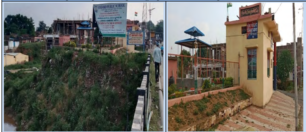
Exhibit 8.6: A police picket constructed at the LW dumpsite, in the Medininagar Municipal Corporation (photograph taken on 20 September 2022)
