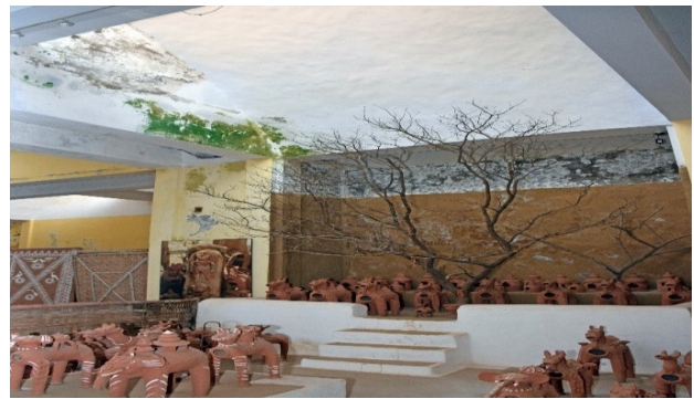
Mosses at the wall
