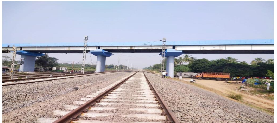
Photo No. 9: Rail Over Bridge
