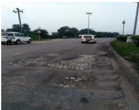
Photo No.13: RD 22.6 km of Sambalpur-Rourkela road
