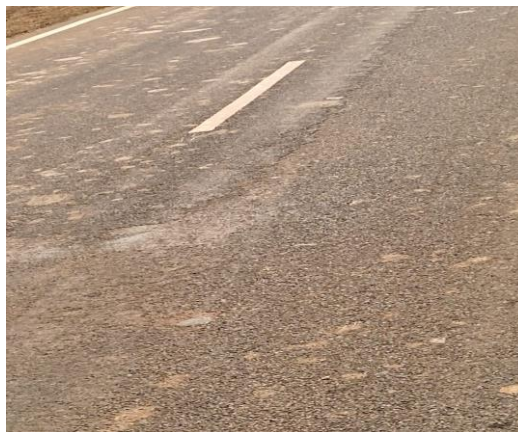
Photo No. 16 : RD 65 km of Sohela-Nuapada road
