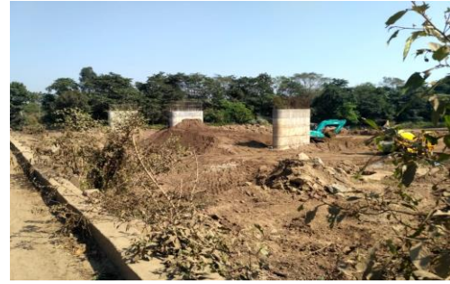
Photo No.11 Construction of Bridge over River Mudra
