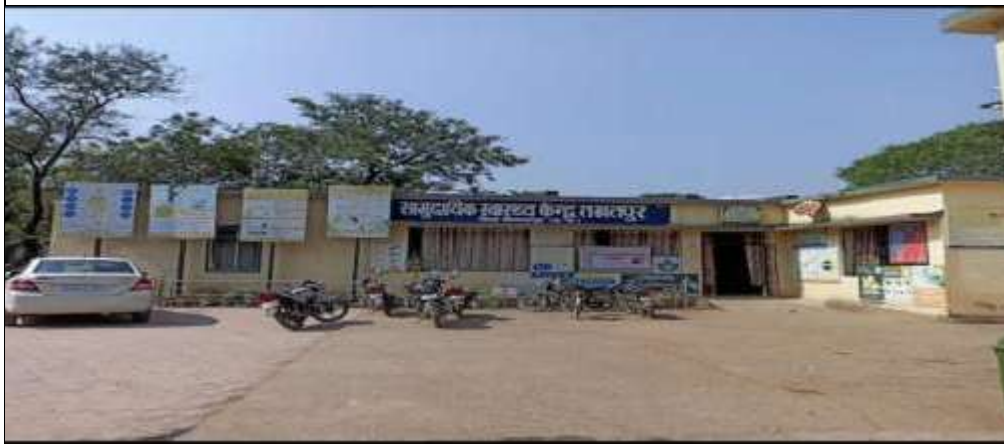
4: CHC Takhatpur running in PHC building (Date 22.03.2022)
