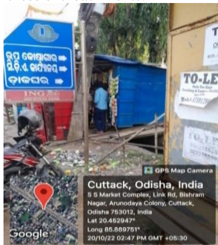
Photograph 30: Shops over drain, in front of CDA Office, Cuttack
