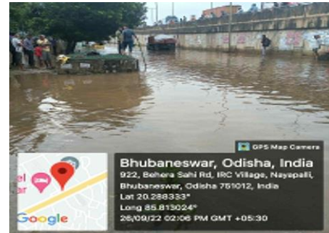
Photograph 15: Water logging at Fly over bridge near ISKCON temple Bhubaneswar
