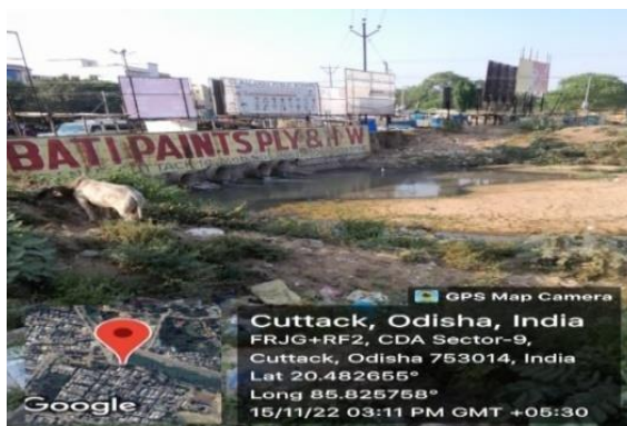
Photograph 38: Sewerage outfall into Petta Nallah, in CDA area
