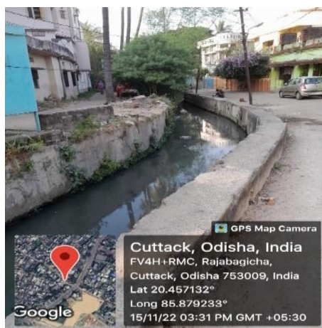
Photograph 23: Drain without cover slab near Rajabagicha Cuttack
