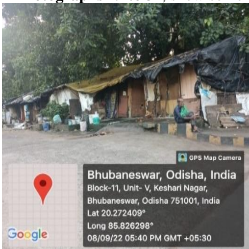
Photograph 29: Construction of houses over drains, near EIC (Civil) Office, Bhubaneswar
