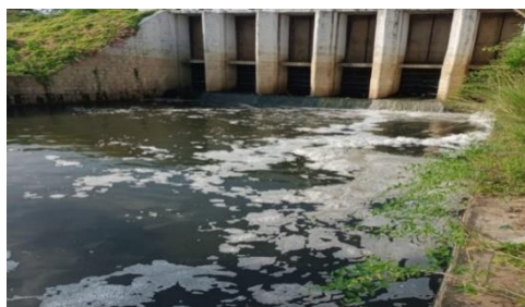
Photograph 27: Outfall of Dhobijore nallah into river Mahanadi, due to non-completion of the sewerage project
