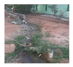
Photograph 3.1.11: Accumulation of waste water, due to partly constructed drainage system at the STGH, Tikabali HS, Tikabali Block, Kandhamal District
