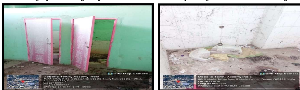
Photographs showing dilapidated condition of sanitary fittings installed in the building
