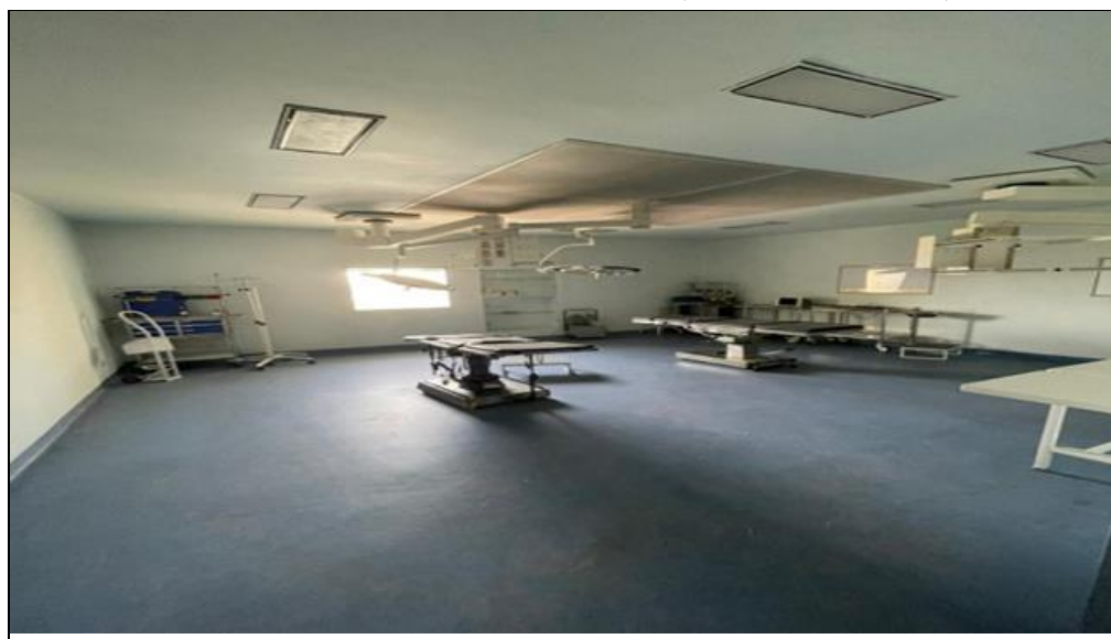
Non-functional OT at SDCH Samalkha (as on 06 March 2022)
