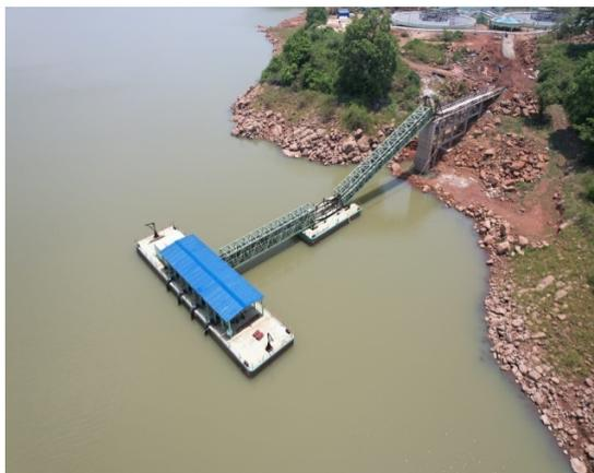
Picture-6: Floating jetty type intake well
