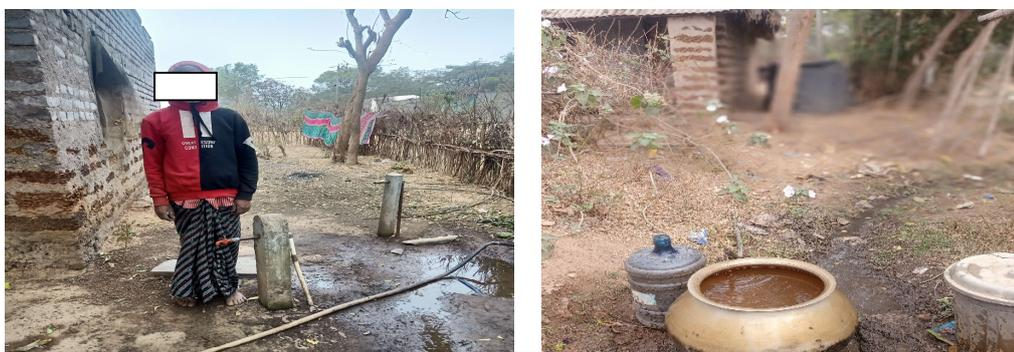
**Picture- 3 and 4:** Leakage and broken tap of the households at Mithigaon Village of Hatadihi block
