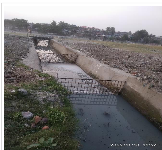
Fig 4.24: Gratings installed in a drain falling in River Mahananda to arrest Solid waste
