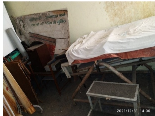
Labour room of Sub Centre Harrayala, Dehradun was being used as store room
