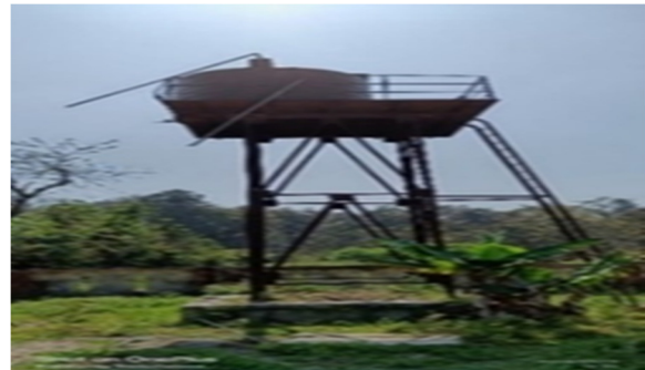
Incomplete overhead water tank, in PHC, Chakalua, Nainital
