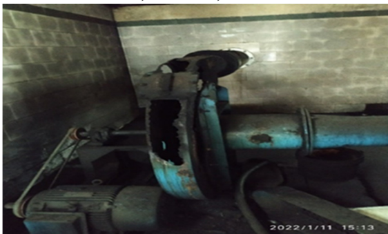
Out of order burnt toxic gas exhaust in CBWTF Haldwani, Nainital
