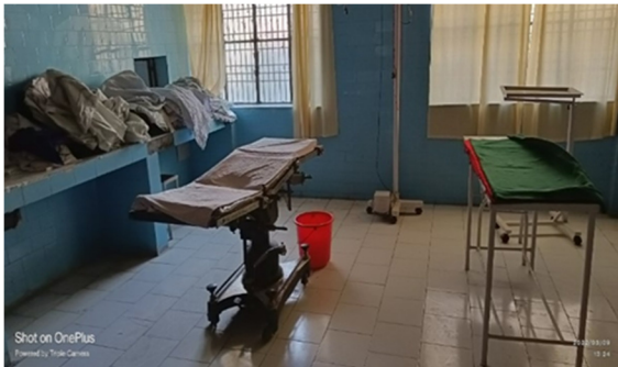
Unequipped OT was being used as clean linen storage at CHC, Kotabagh, Nainital
