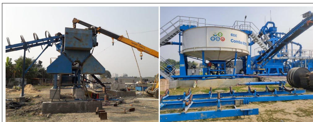
Fig 4.14 & 4.15: C&D Waste Processing Plant under construction at Pathargata
