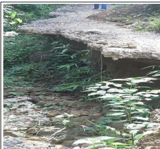
Photograph 4.2.5: The last stretch of the approach road leading to the steel foot bridge which was washed away by first rain
