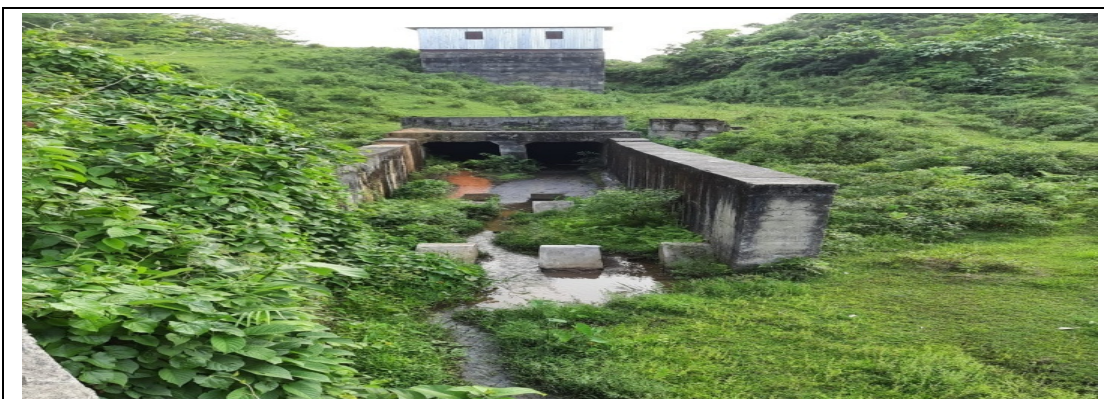
Photograph 3.4.3: Seepage of water through Steel gate control room and under sluice at downstream side
